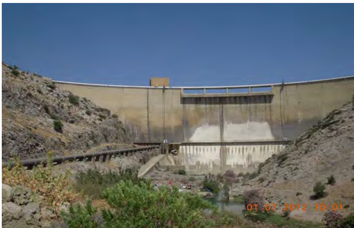
Photo 2. Hydro electricity Generation
