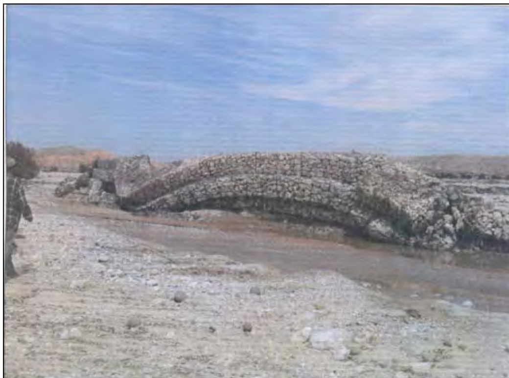
Photo 7. Flood Event in September 2009 in Redeyef –Gafsa (Destruction of works of water and soil conservation in Tarfaoui river)
